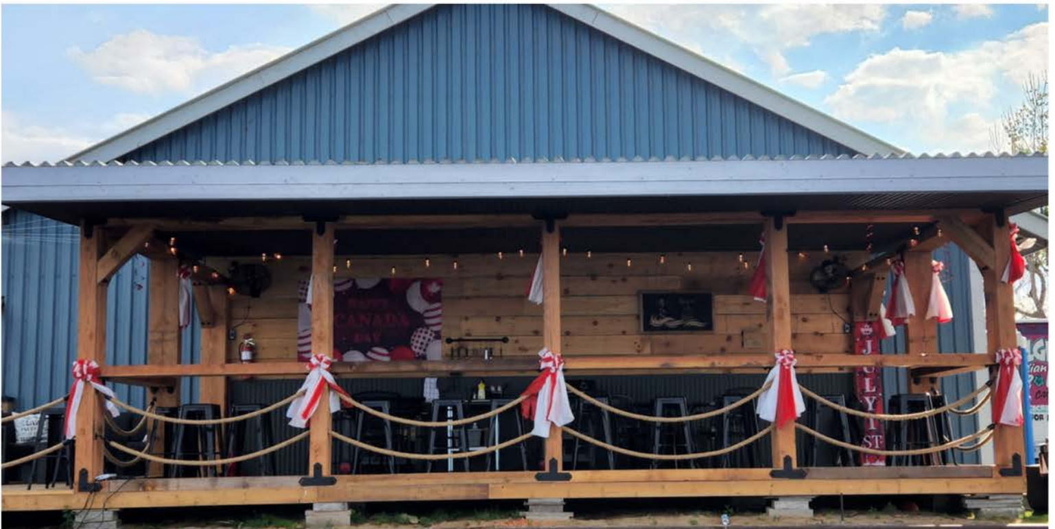
40' x 15' Douglas Fir Dockside Pavilion
